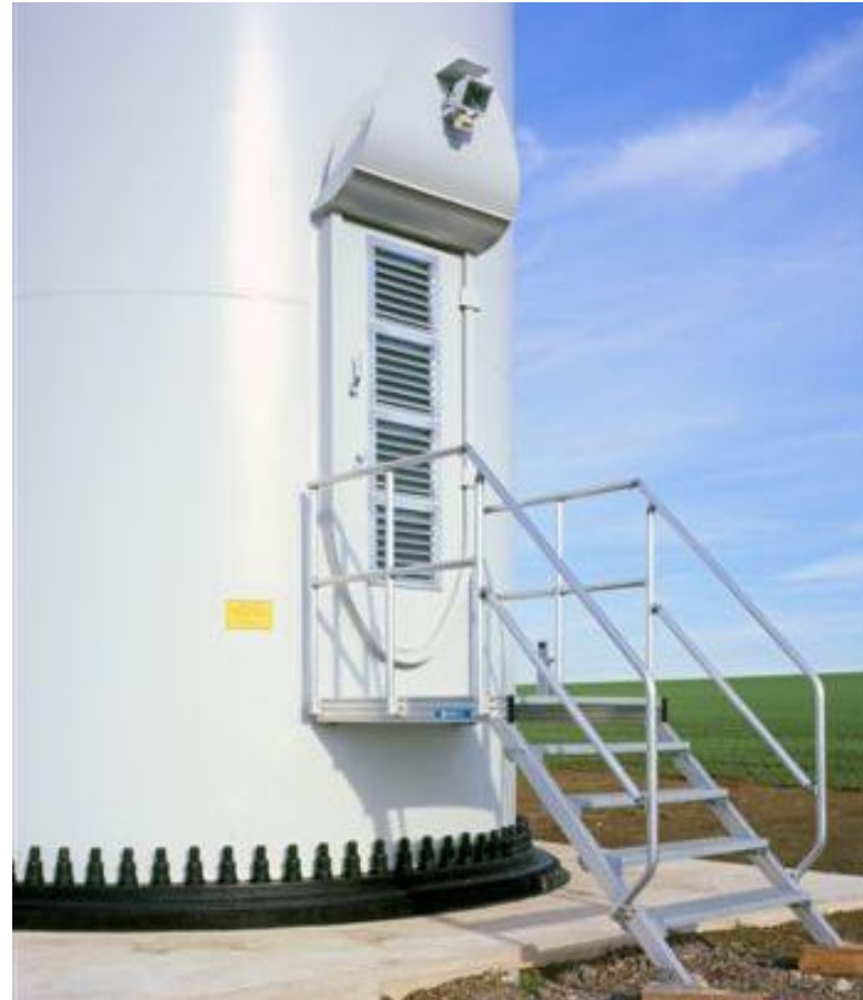
Tower access stairway
